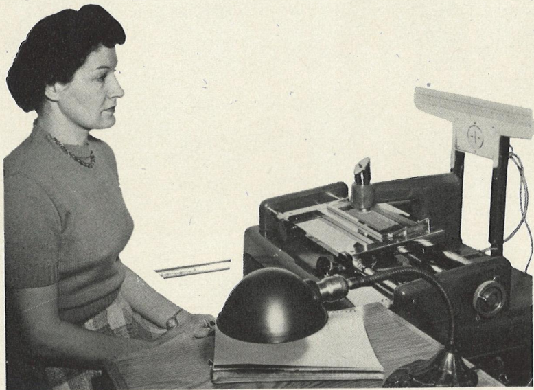
ANN SHAW AT THE DENSITOMETER , which helps interpret spectrographs taken of ore samples. If line in spectrum is heavy, large amount of element is present.
